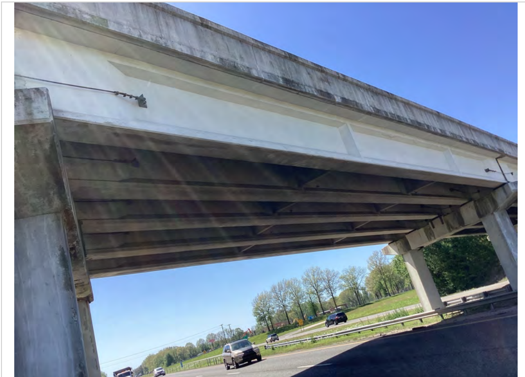
Span 2 bottom deck
