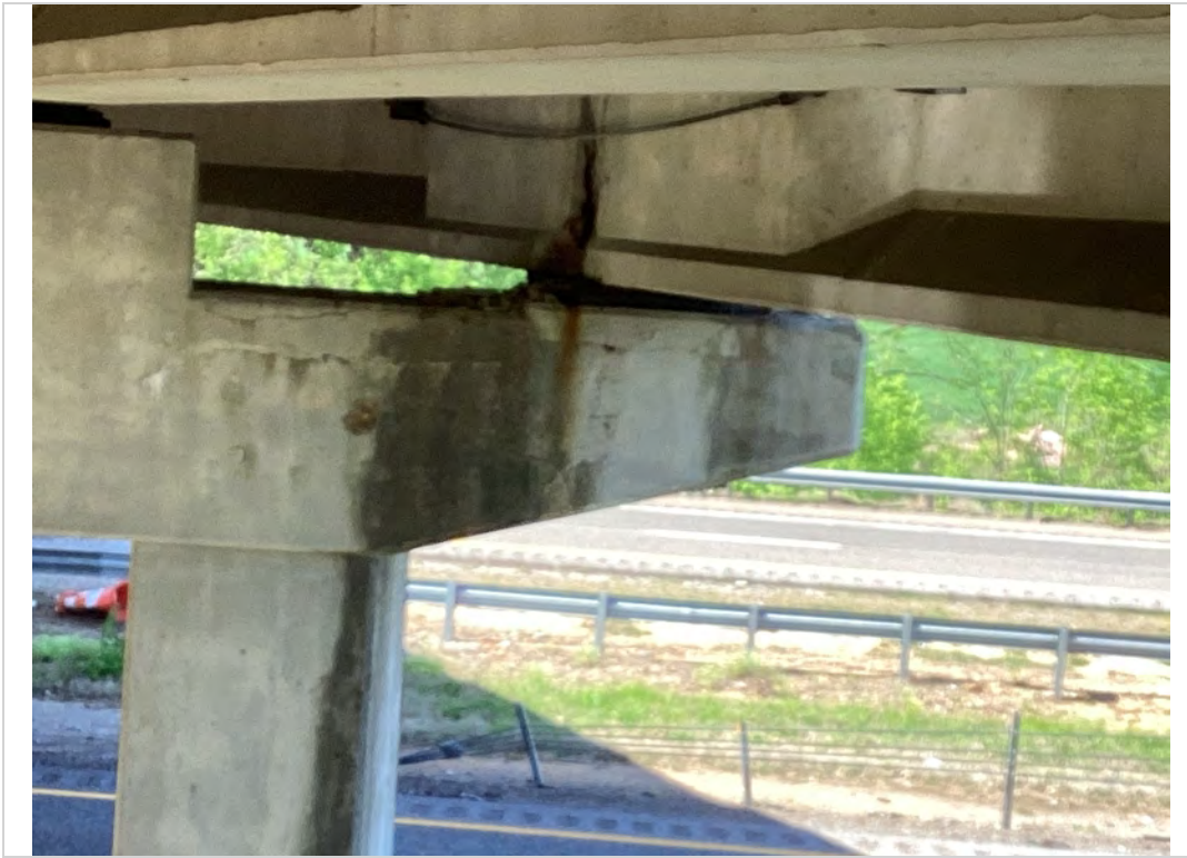
Bent 1 bearing E spalled to steel
