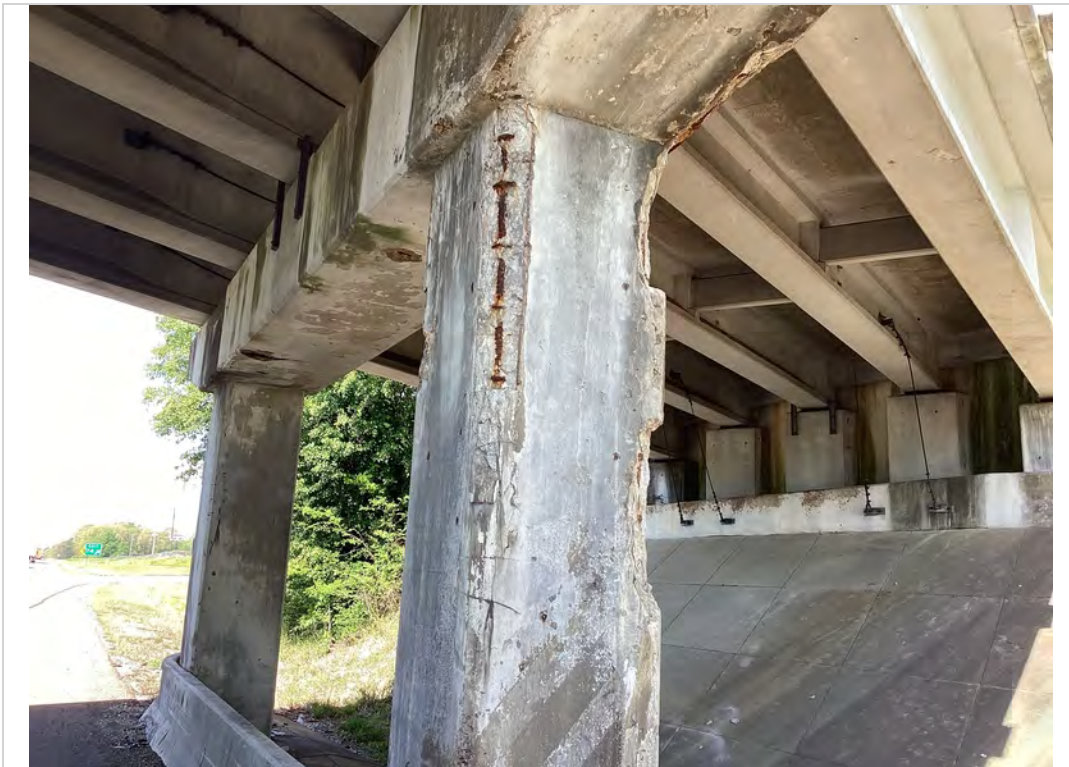
Bent 3 column b
