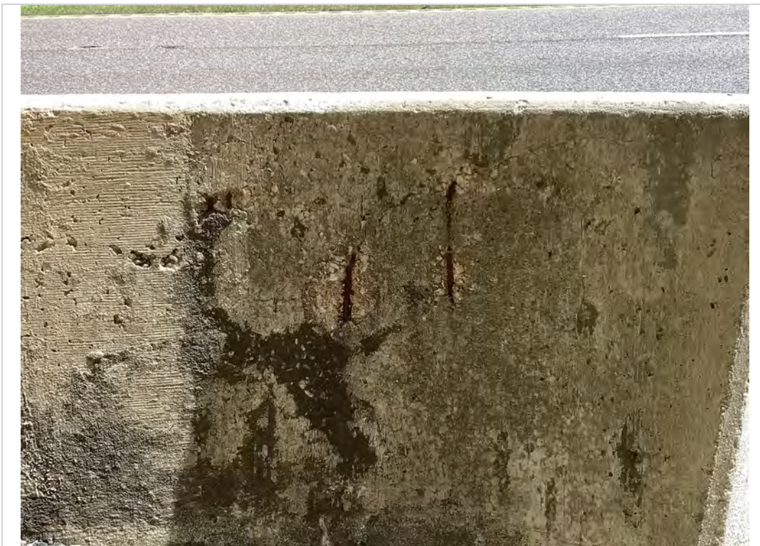
Bent # 3 crash wall/ parapet , surface steel area(s)
