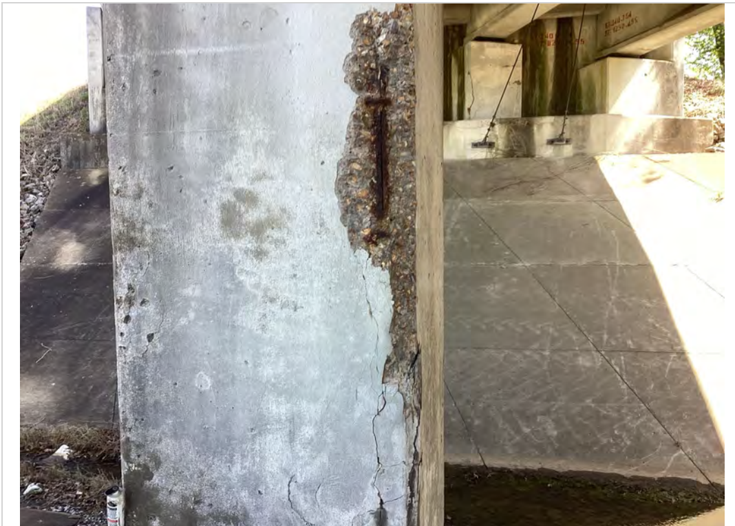
Bent 1 Pile B rear side
