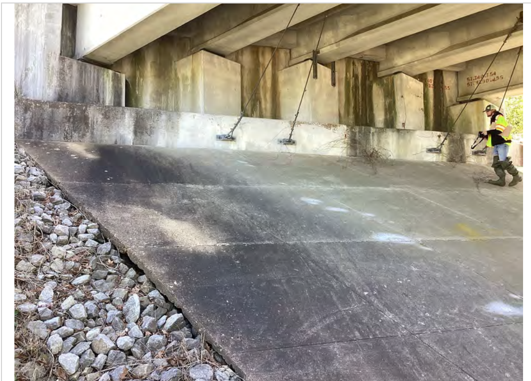
Abutment 1 looking back
