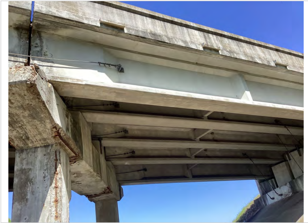
Span 1 bottom deck
