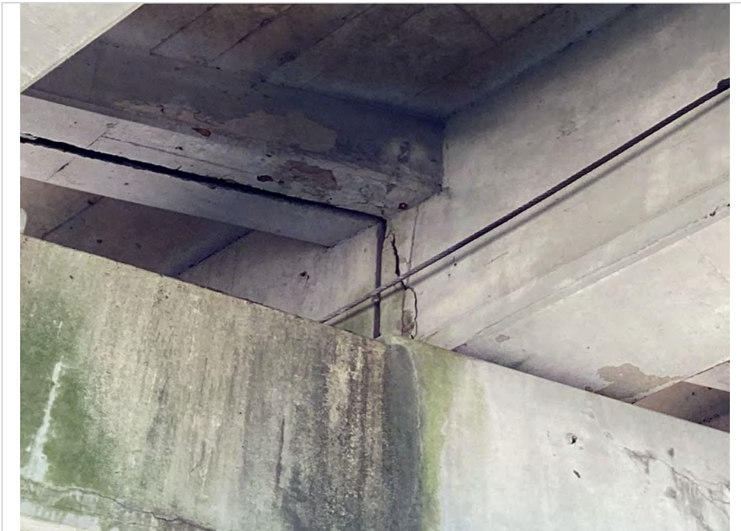
Span 2 beam d
